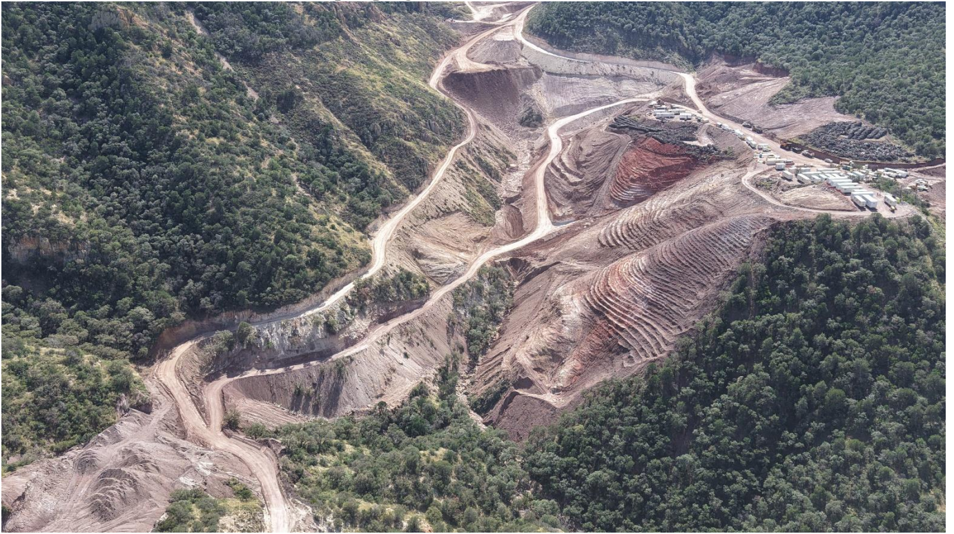
Photo 3: Earthworks of the waste dump in progress
