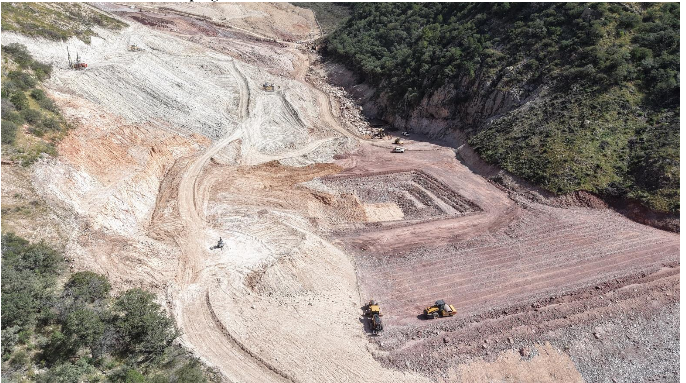
Photo 4: Ponds earthworks in progress.
