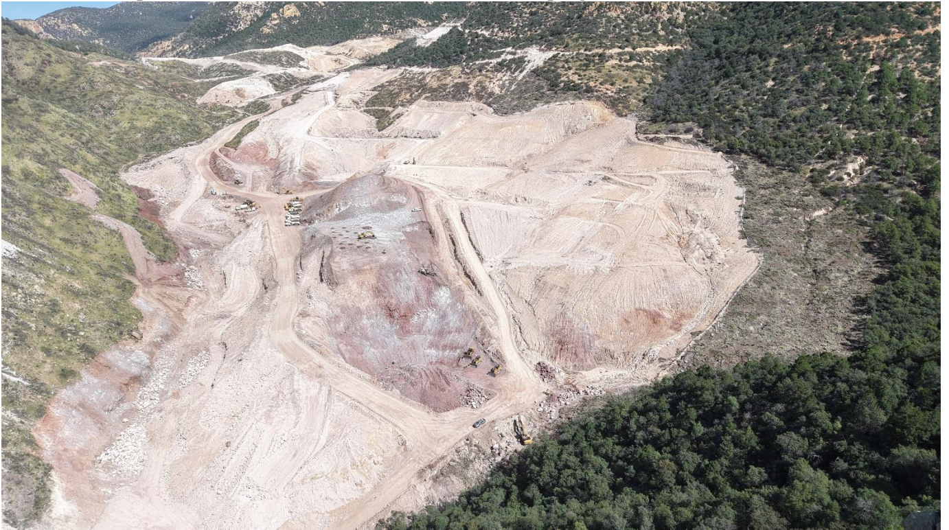
Photo 1: Leach pad and mine facilities area with earthworks in progress
