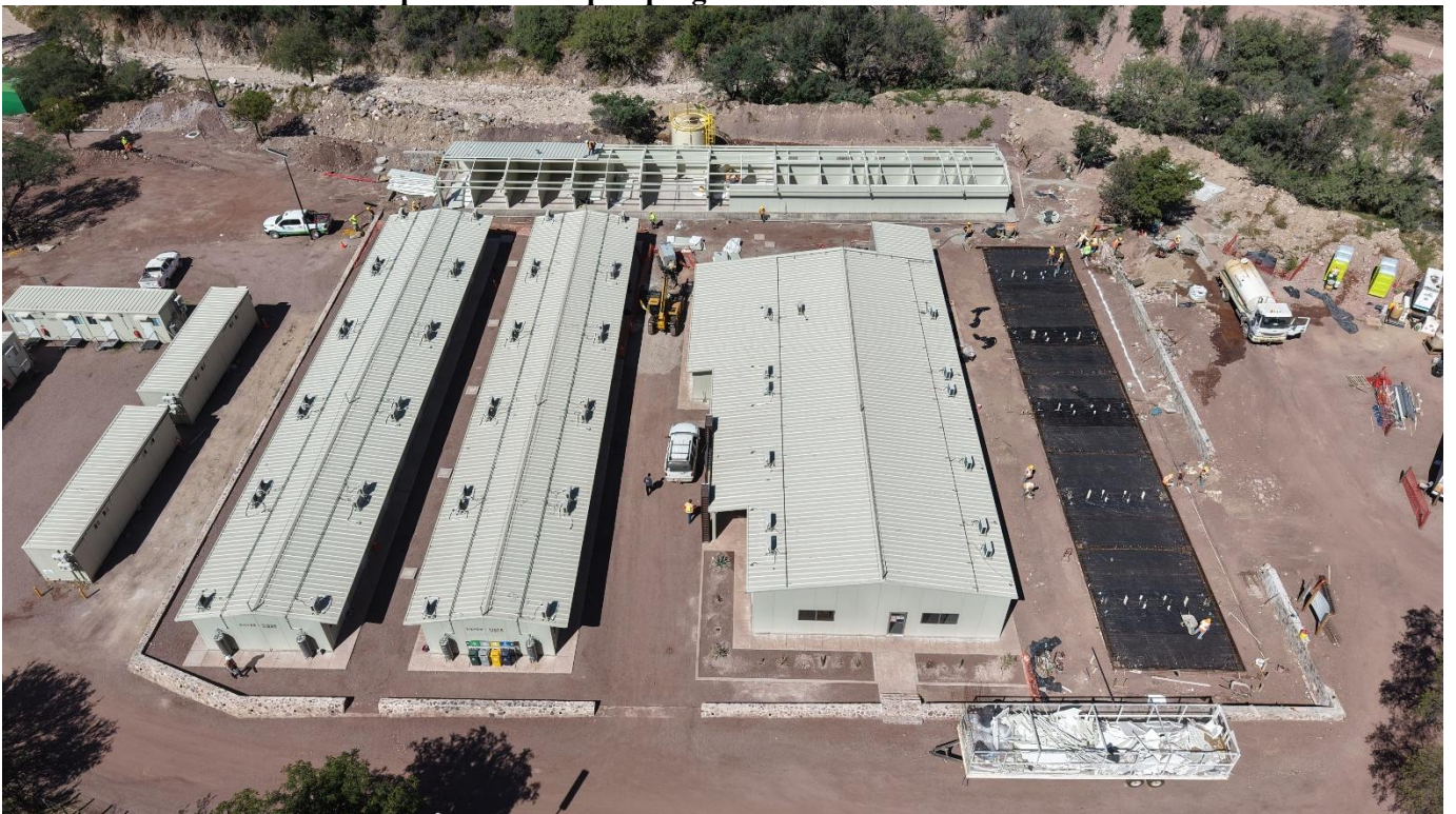
Photo 2: Construction of the operations camp in progress
