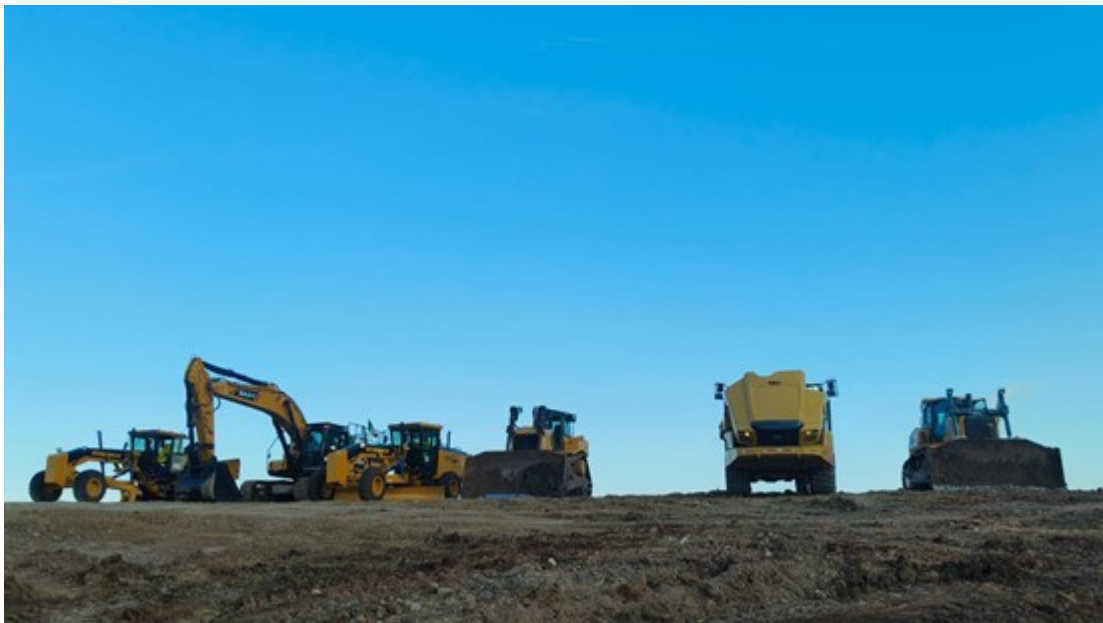
Figure 2 – Construction Equipment on Site
