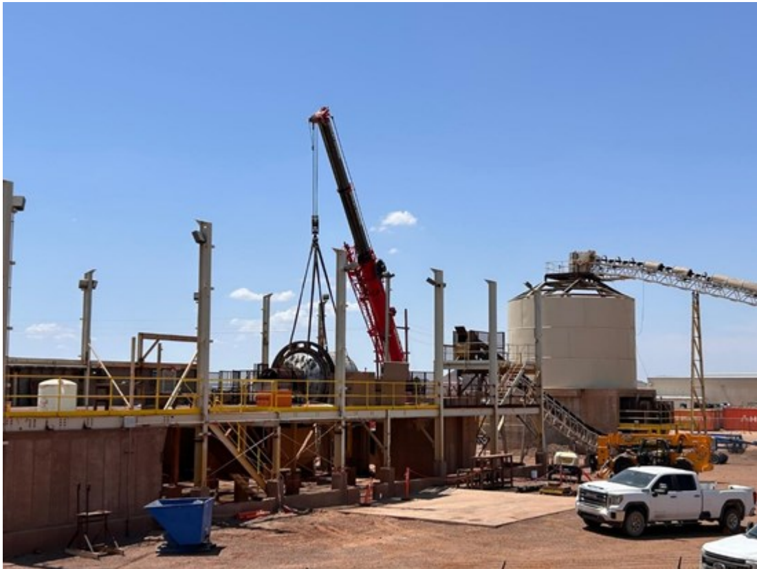
Figure 1. Historic ball mill being removed from the process plant
