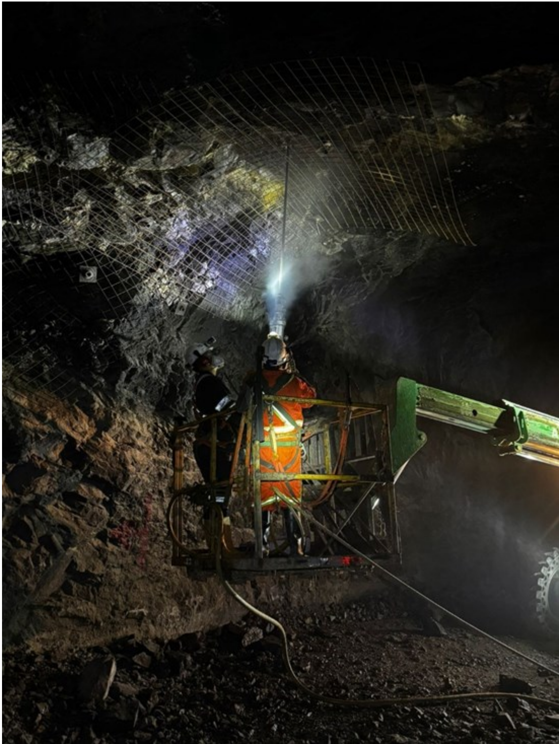
Figure 3: Installation of Ground Support at Promontorio
