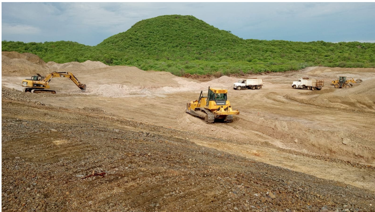
Photo 1: Recent work at the Pilot Facility as the heap leach pad is near completion.
