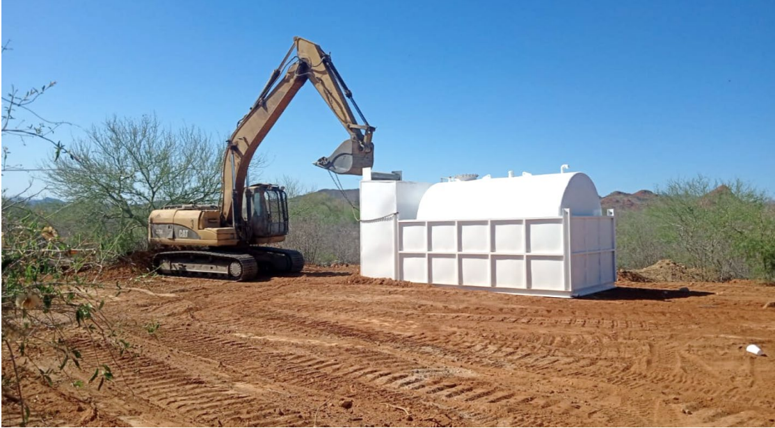
Photo 3: Onsite fuel storage for pilot equipment and drilling.
