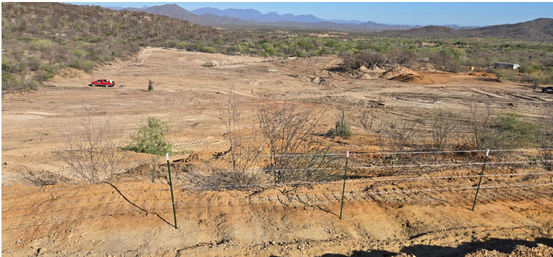
Photo 1: 6-hectare area cleared for permitted 10-year pilot facility.
