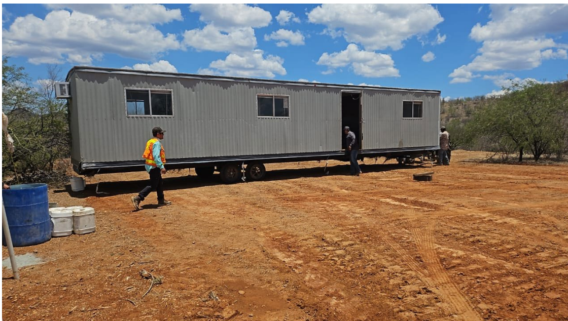
Photo 2: Onsite office installation.
