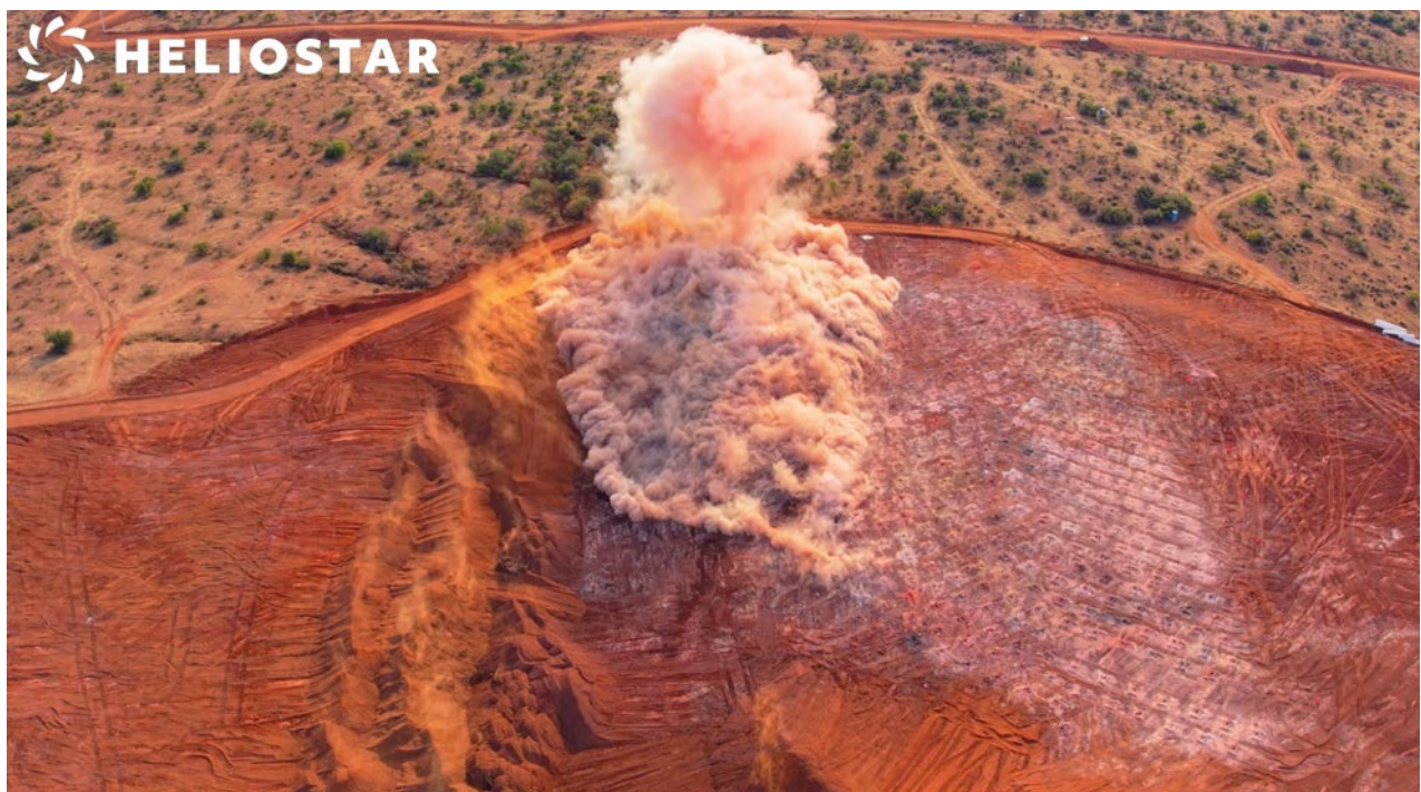
Figure 2: First blast of the Corner Area at San Agustin
