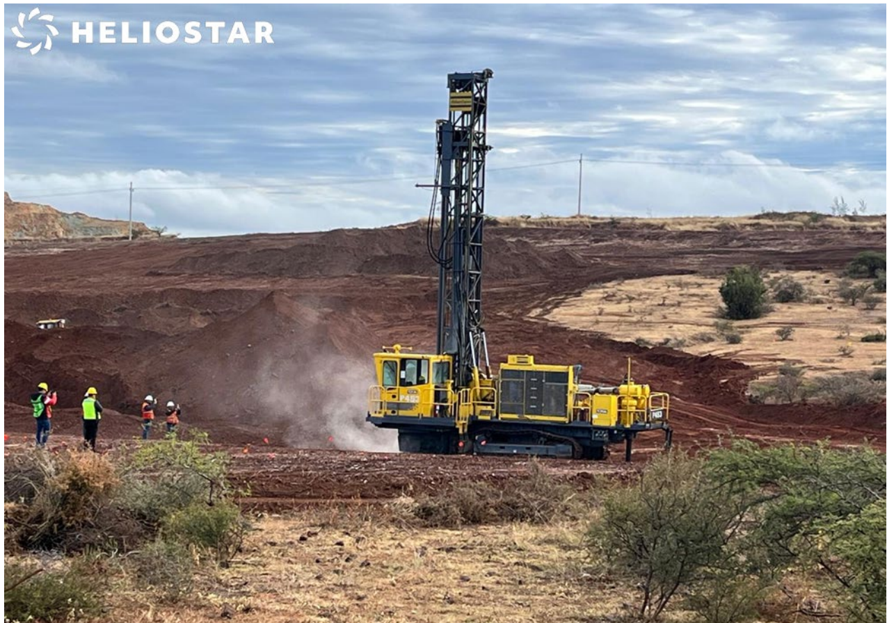
Figure 1: Production drill rig drilling blast hole pattern in Corner Area at San Agustin
