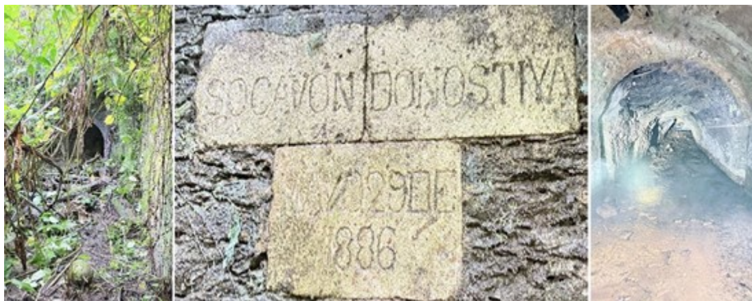
Figure 2: Historic Mine Portal
