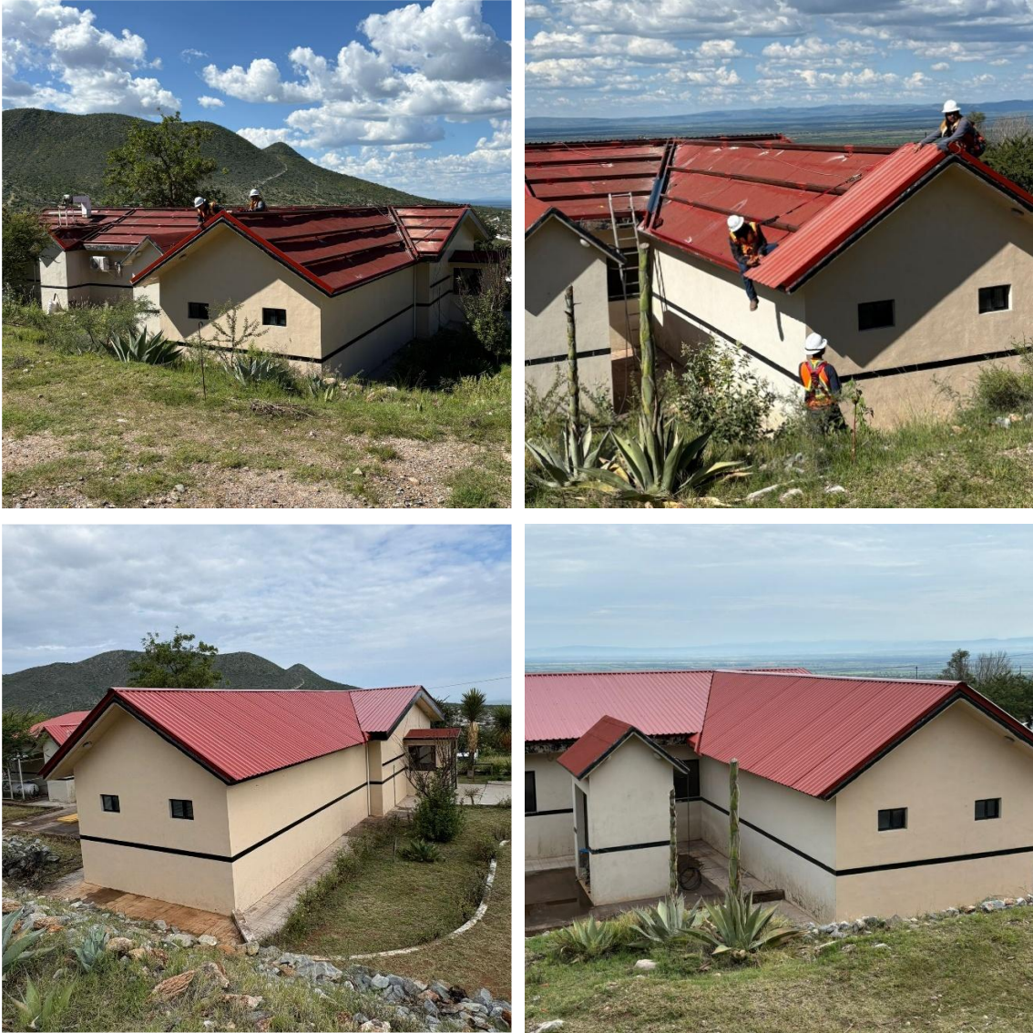
Figure 1 - Roof Replacement on Kitchen and Mess Hall
