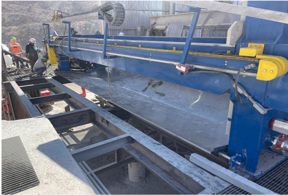
Image 1 – New Tailings Filter Press being installed at Tahuehueto
