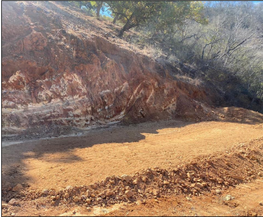
Figure 3. New drill pad ready for rig mobilization on Diamante 1.
