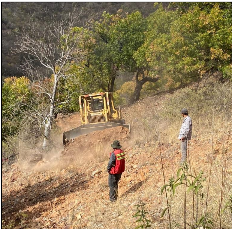
Figure 2. Colibri geologist provides direction to equipment preparing trail and drill pads at Diamante 1.
