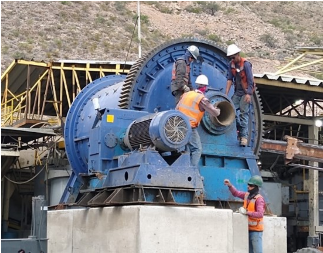
Photo 1. Ongoing Work at Plomosas Mill
