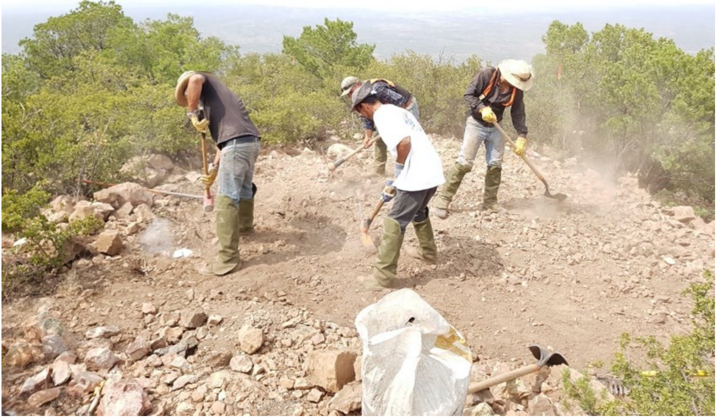
Figure 2a: Drill pads being built and trails widened
