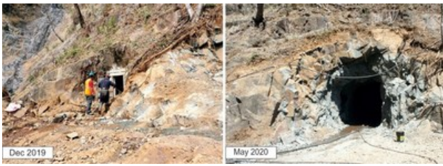
Figure 5: San Marcial Tunnel - Underground Development in 2020 (CNW Group/GR Silver Mining Ltd.)
