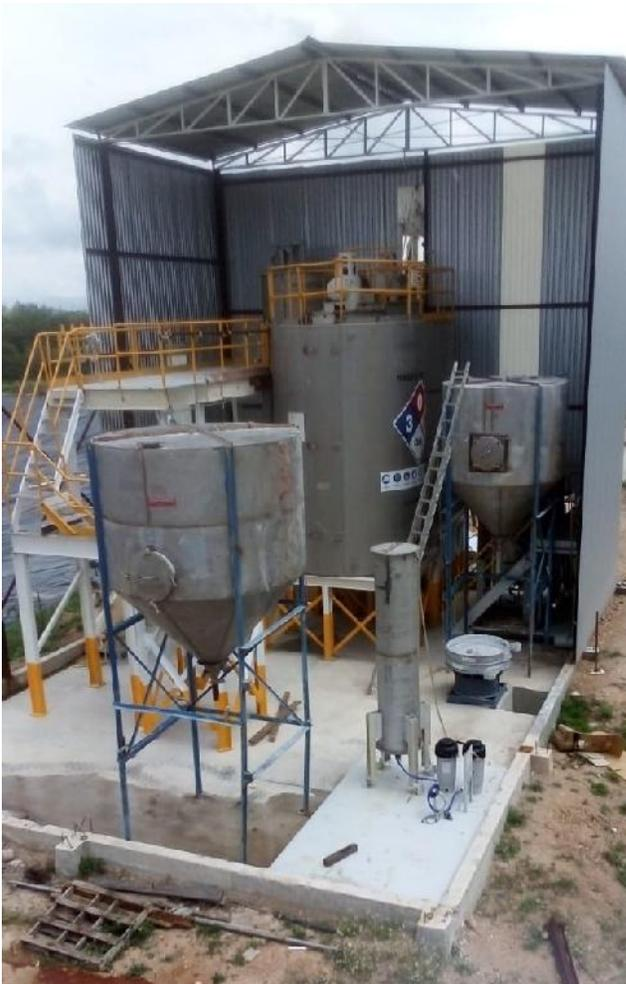
**Leach plant with all major equipment installed and ready for testing**
