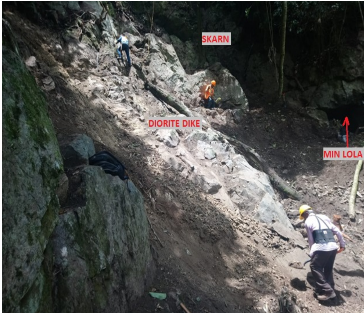
Figure 3 - Overburden Stripping at La Lola Mine
